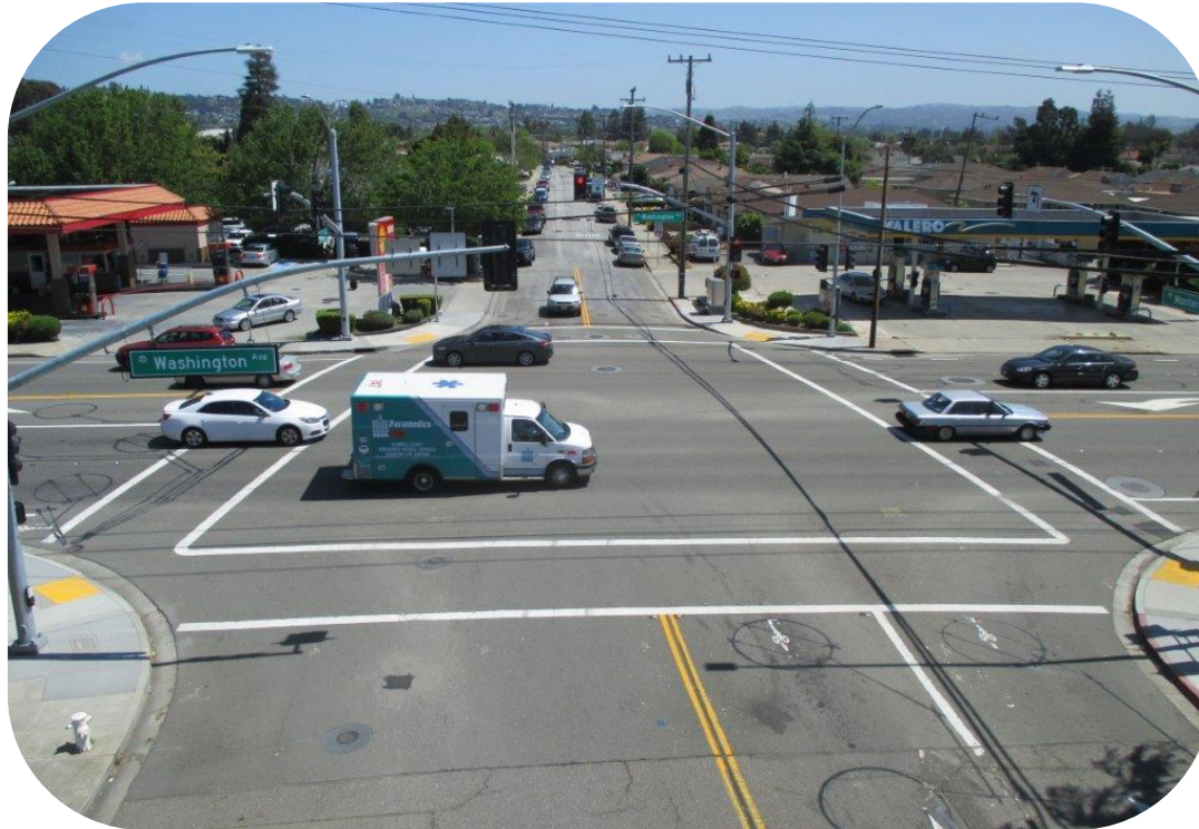
Aerial View From Monterey Boulevard looking East of Improvements Including New Mast Arms, Signage, Safety Lighting and Designated Left Turn Lanes on Washington Avenue
